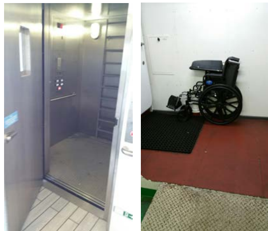
Elevator buttons high contrast and tactile. Operator wheelchair available on vehicle deck. Elevator has a ramp for easier access on vehicle deck. Handrails should be on each elevator wall
