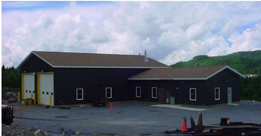
New Highways Depot in Corner Brook
